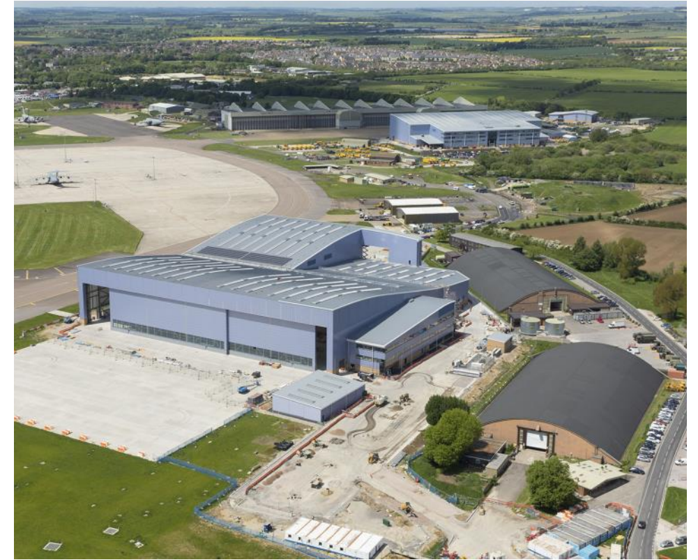
Photo 7. Aerial view of Atlas hangar
